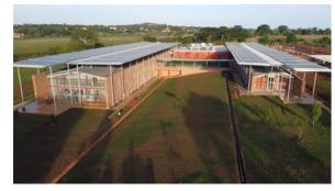
construct the hospital's walls sustainably while, at the same time, guaranteeing versatility and durability. The use of such a widely available material as clay reduced the project's environmental impact and fitted in with local tradition.
